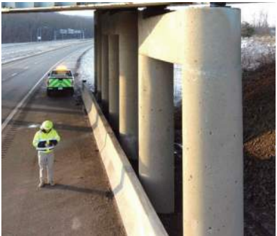
4 Piers | Round column, pier cap, concrete
