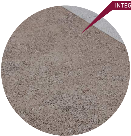
TOP-SEEDED INT. COLOR CONCRETE Cycletrack
