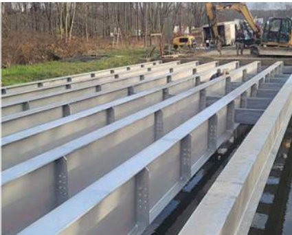
2 Steel girders | Galvanized steel
