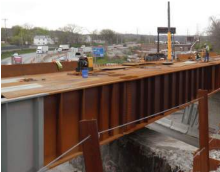
3 Steel girders | Weathering steel
